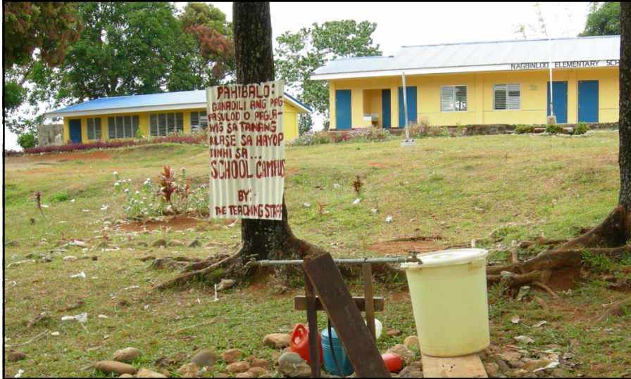
Two additional school buildings completed in May 2005 with the school water standpipe in the foreground.
